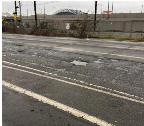
**Figure 8:** Deteriorated Roadway Conditions on East Marginal Way S
